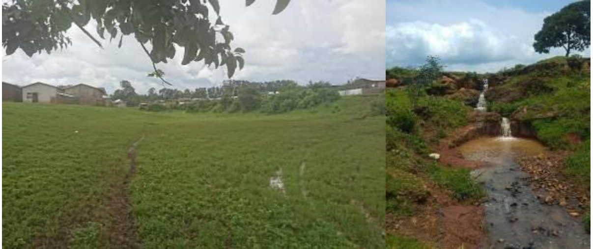
Figure 8-20: Show the upstream and midstream view of the drainage line 1 running through the site
