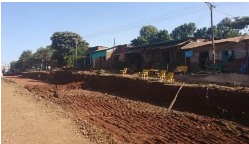
Figure 8-38: Current upgrade activities of the Federal Highway No. B_31 within Motta
