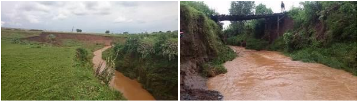
Figure 8-19: Photos showing the Yiser River to the west of the IAIP (Source: ESIA team site investigations)
