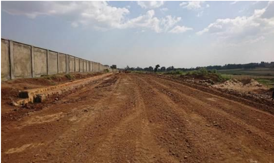
Figure 8-43: Alternative road along the western boundary of the IAIP
