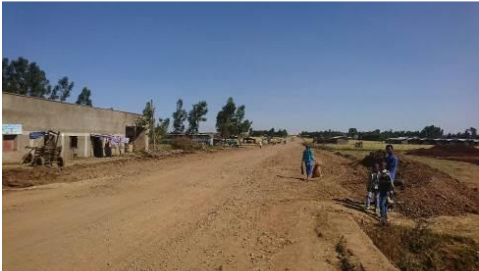
Figure 8-37: Image federal highway no.B_31 (Source: ESIA team site investigations)
