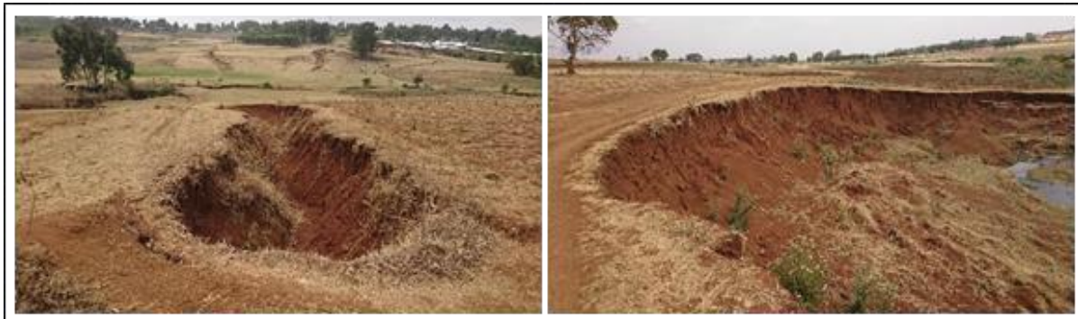
Figure 8-2: Erosion along the western boundary of the IAIP site
