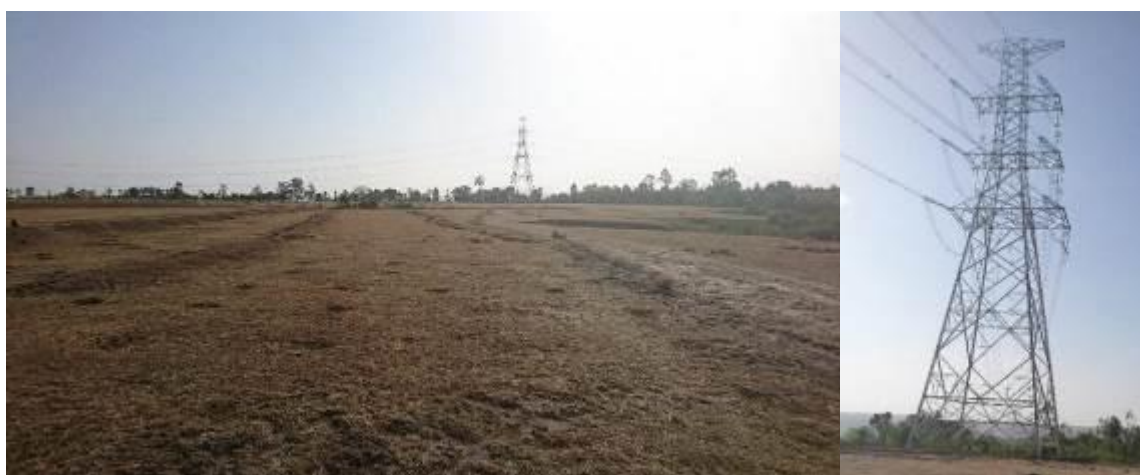
Figure 8-44: New overhead power line structure on site
